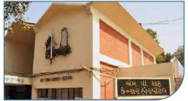
M. P. Shah Cancer Hospital Civil Hospital Campus, Ahmedabad
